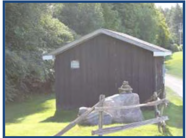
PUMP HOUSE (HOLE #7)
