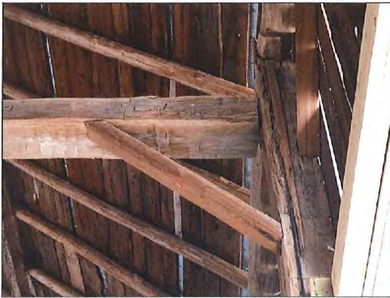
Photograph 08 - Beam-Post Connection - Separating
