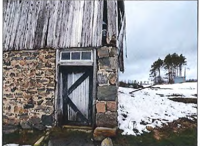
Photograph 13 - Rubble Stone Foundation Wall - Void Mortar Joints
