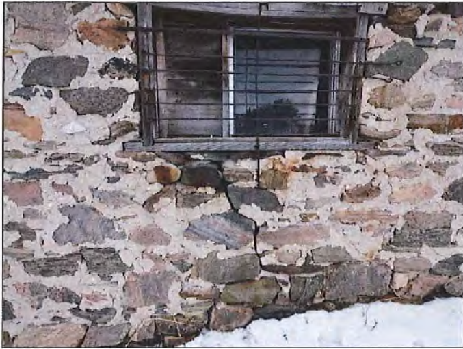
Photograph 14 - Rubble Stone Foundation Wall - Crack
