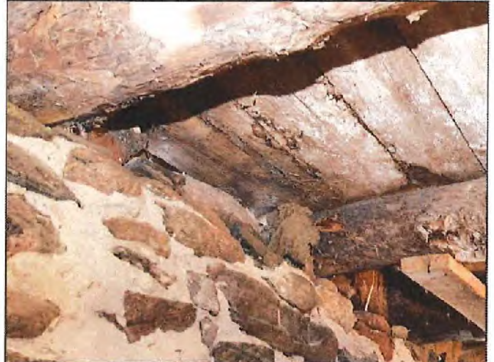
Photograph 11 - Upper Level Floor Purlins
