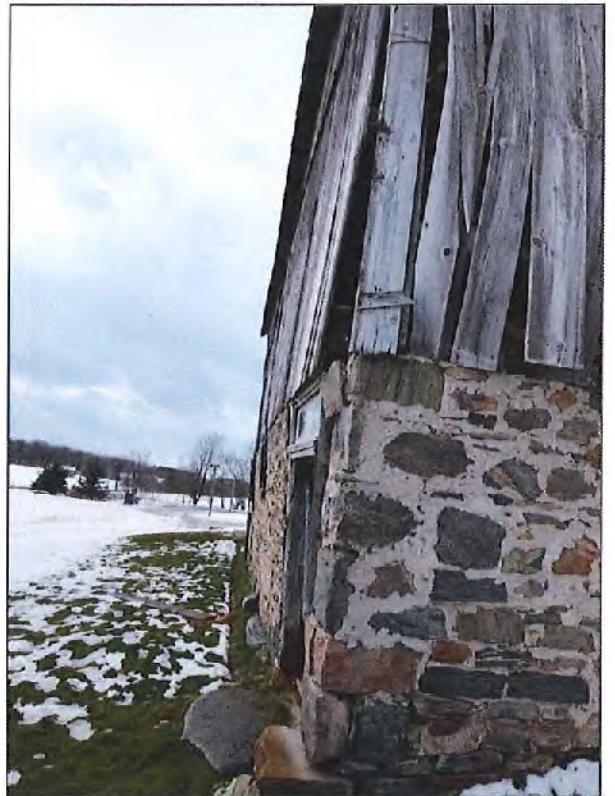
Photograph 09 - East Foundation Wall - Leaning
