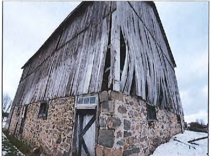
Photograph 03 - Damaged Wall Boards - North Wall
