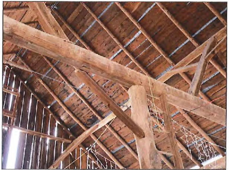
Photograph 05 - Knee Brace - Connected One End Only
