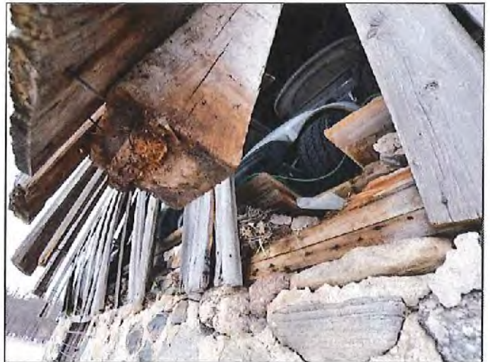
Photograph 15 - Post Base - Rotten Tongue
