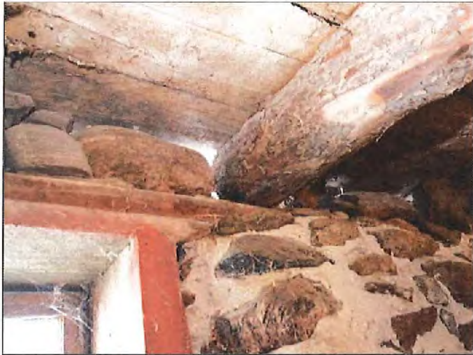
Photograph 10 - Upper Level Floor Purlins
